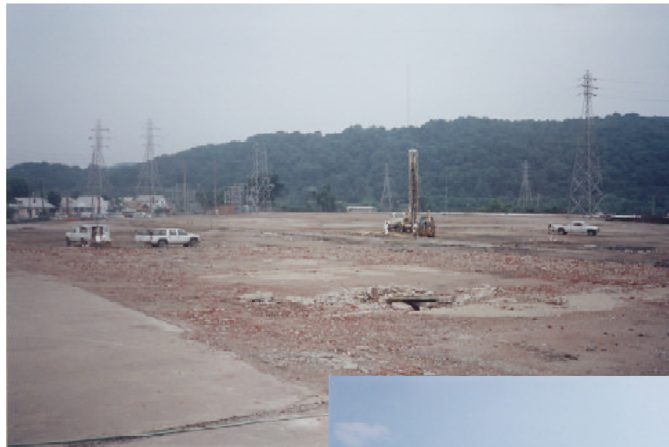
Left: Crews arrived on the former FMC East Plant site in the last week of July 1998 for the final phase of surface and subsurface soil investigation.
